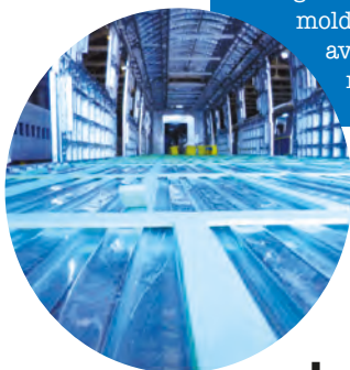
BELOW: Sylomer strips integrated in a floating floor
